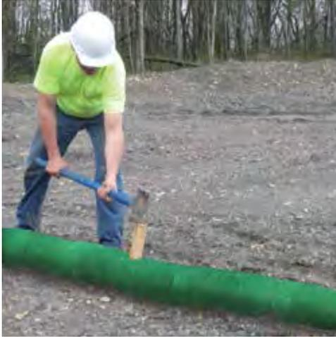
SiltSoxx do not require any trenching or soil disturbance. Simply stake them in to the ground. SiltSoxx can also be used on pavement or frozen ground.
